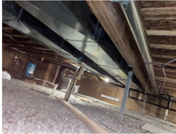
Figure 3 – Ductwork Mains Installed (2)
