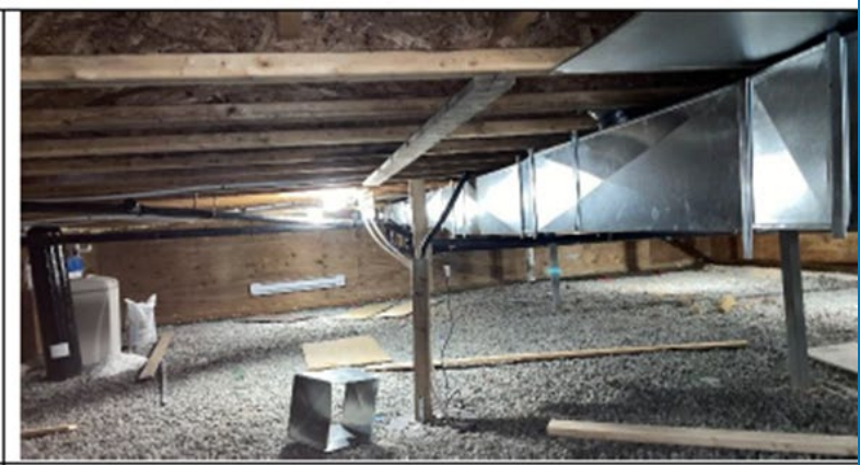
Figure 2 – Ductwork Mains Installed
